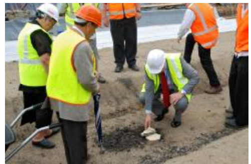
CEO Geraint Martin places a piece of the old building in the ground.
