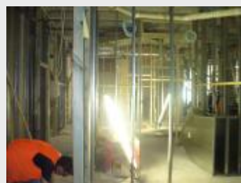
Walls are being constructed.
