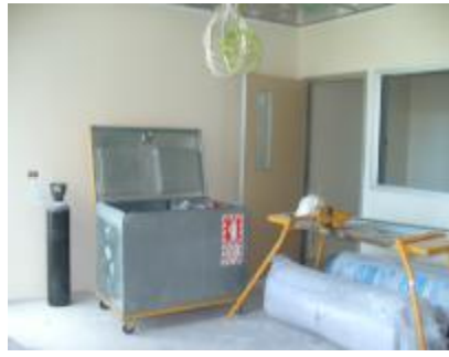
Positive pressure Isolation/Ante Room
