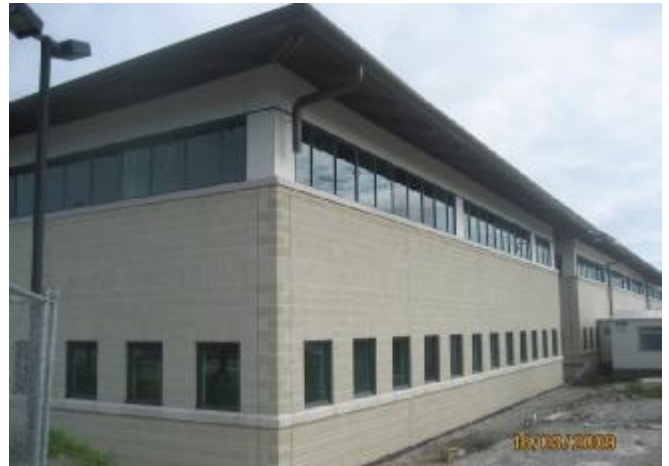
Building A - with the scaffolding recently removed
