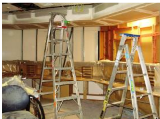
The new reception takes shape
